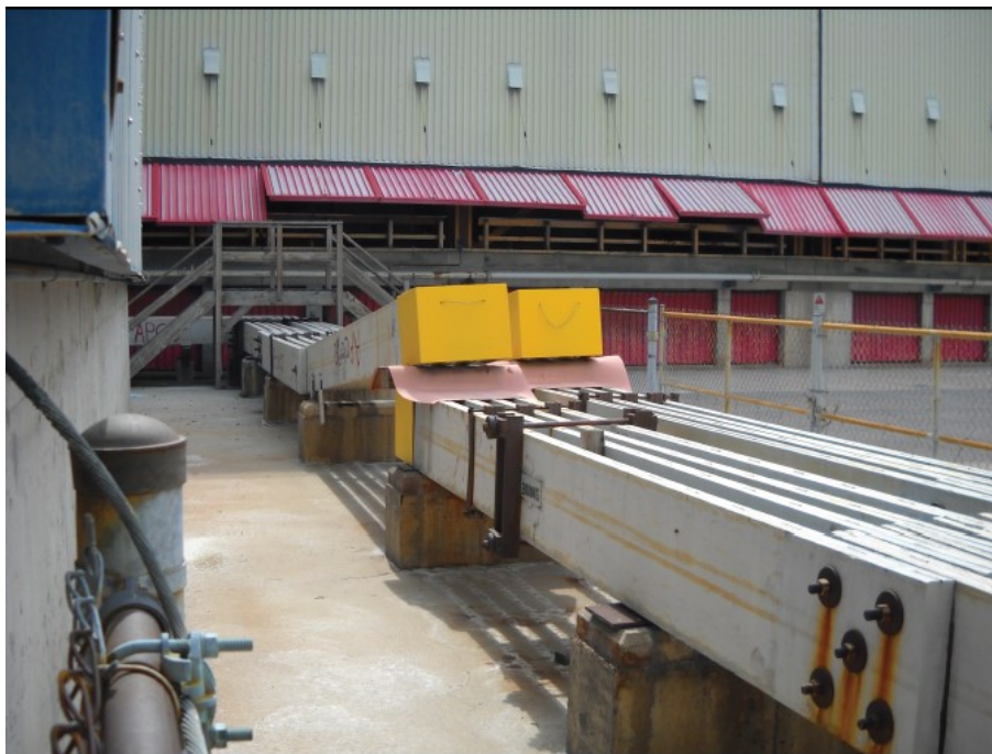
Figure 18. Half-potline by-pass bridge.
